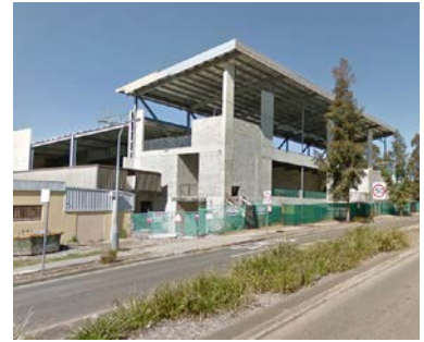
Club facilities under construction at Bonnyrigg Ave/Edensor Rd
