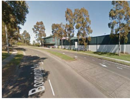
Existing Bunnings site on Bonnyrigg Avenue
