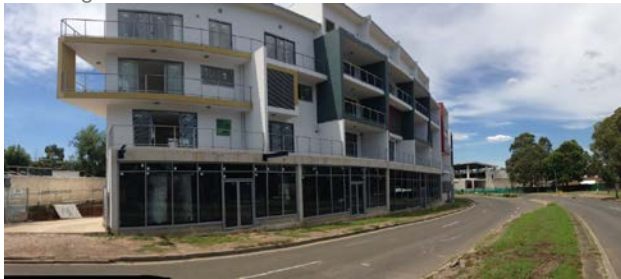
New 6 storey Mixed Use development under construction
